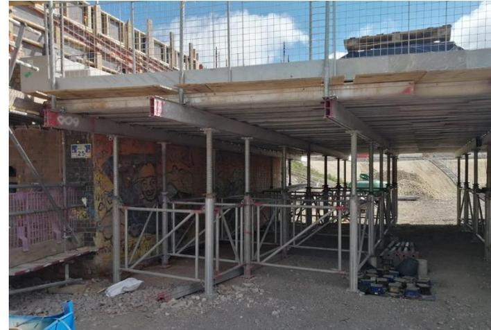
Platform to support the shutters for the concrete
